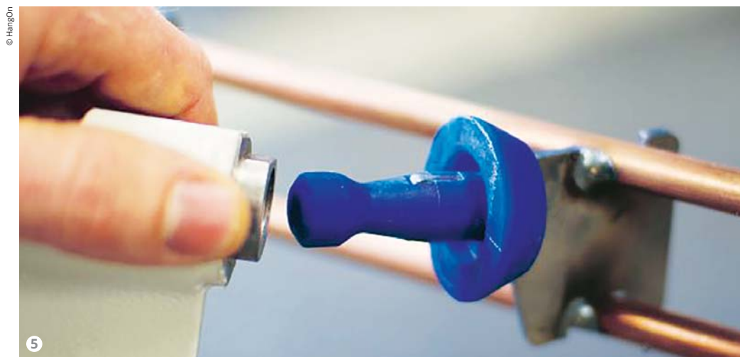
Figure 5: The special GHA Style, masking and hanging system.
